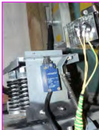
achieve fail safe practices of safety switch design. They incorporate a spring tensioned rope end knock out plate fitted above the compressed spring rope dead-ends, that holds a normally open plunger limit switch closed. Any release of tension on the rope bottles raises the actuating plate thereby releasing the switch to open.
