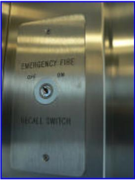
As early as 1930, it was recognised that fire-fighters should be provided with a means of swift access to the upper floors of large buildings. This resulted in conventional passenger lifts being fitted with a break glass switch at the main access floor, that, when operated brought that lift quickly to that floor.
