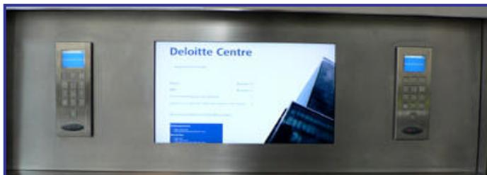
Note the keypad call input design allows users to input the level they wish to go to, and the system screen indicates what lift the user should use, either A,B,C,D etc., relative to the number of lifts in the bank.
