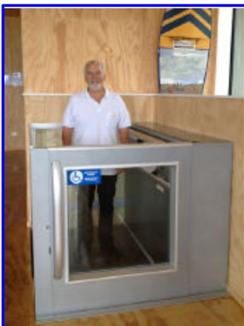
The lift which included automatic swing doors was one of the Cibes A 5000 range of platform lifts which are ideally suited for their small footprint low speed and low ongoing running costs.
