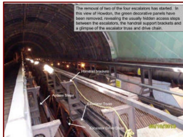
The removal of two of the four escalators has started. In this view of Howdon, the green decorative panels have been removed, revealing the usually hidden access stairs between the escalators, the handrail support brackets and a glimpse of the escalator truss and drive chain.
