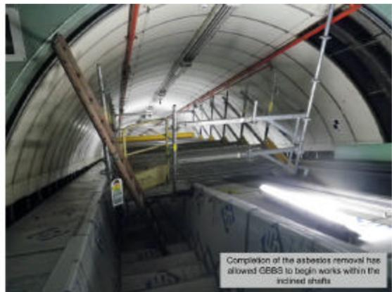
Completion of the asbestos removal has allowed GBBS to begin works within the inclined shafts.
