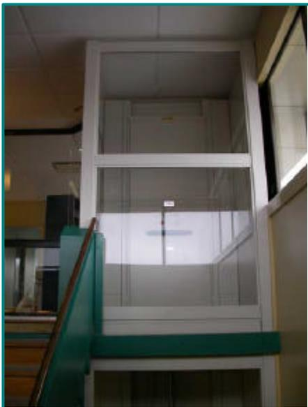
Price ranges up to \$50,000, and the controls require constant pressure on call pushes to operate, but have a soft touch. The internal shaft is flush, fitted with platform edge and overhead non-entrapment sensors that provide total passenger safety.
