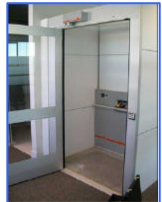
clear the opening door. This also enables sufficient space for exiting wheelchair users to pass. All doors should have vision windows or glazing at a height suitable for wheelchair users to be able to confirm their clear path.
