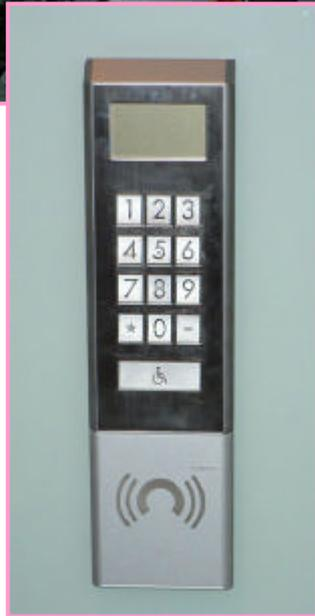
The station consists of a keypad much like the prolific telephone key pad but also incorporates a small display screen. The key pad is to input the floor you wish to go to, and the display indicates which lift to use.
